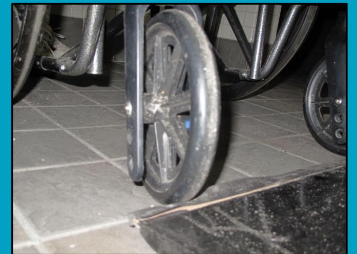
Make ramp insert between the ramp holder more secure and achieve minimal gaps
